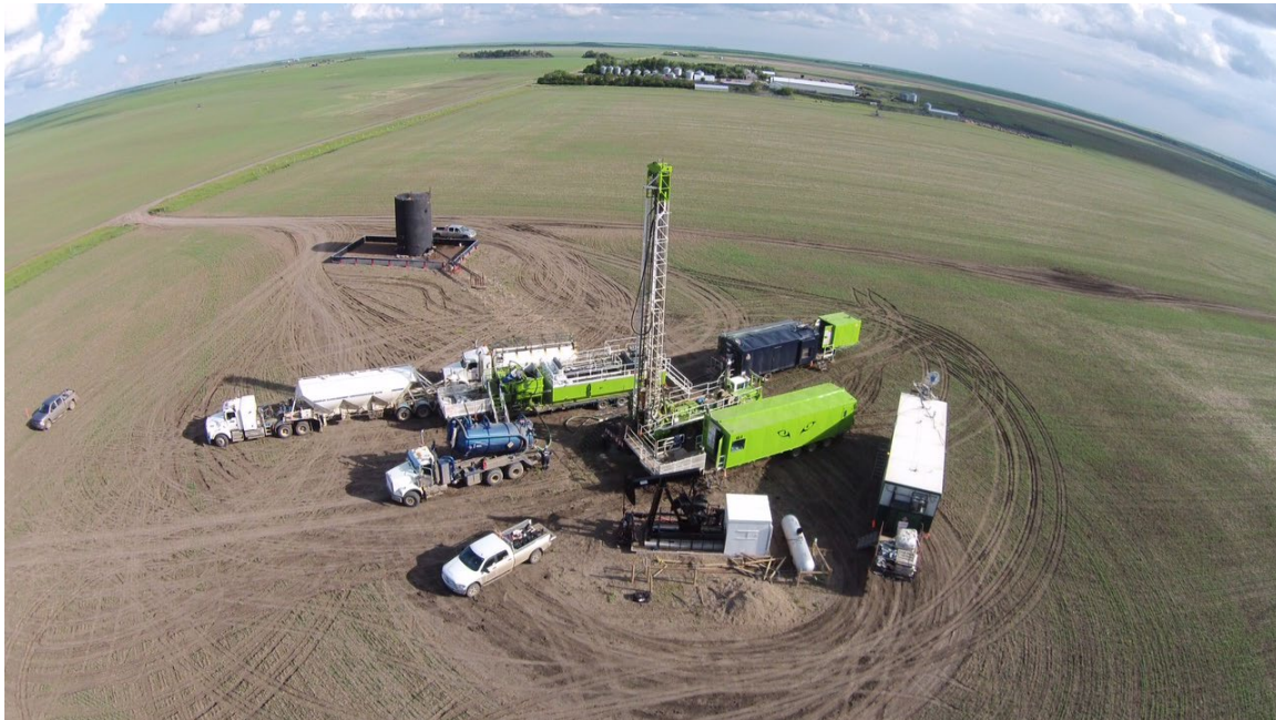
Figure 16-19: Pre-Set Drilling Rig Field Photo Example
