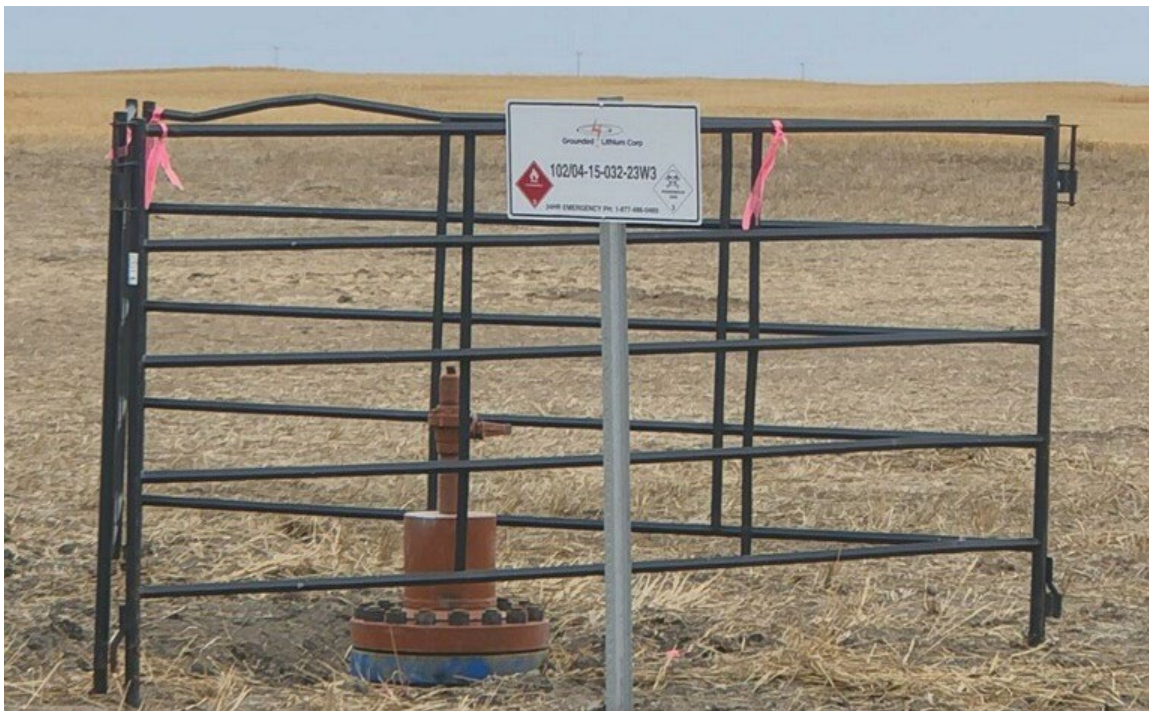
Figure 2-1: Surface Site and Wellhead (GLC 102/04-15-032-23W3/00)
