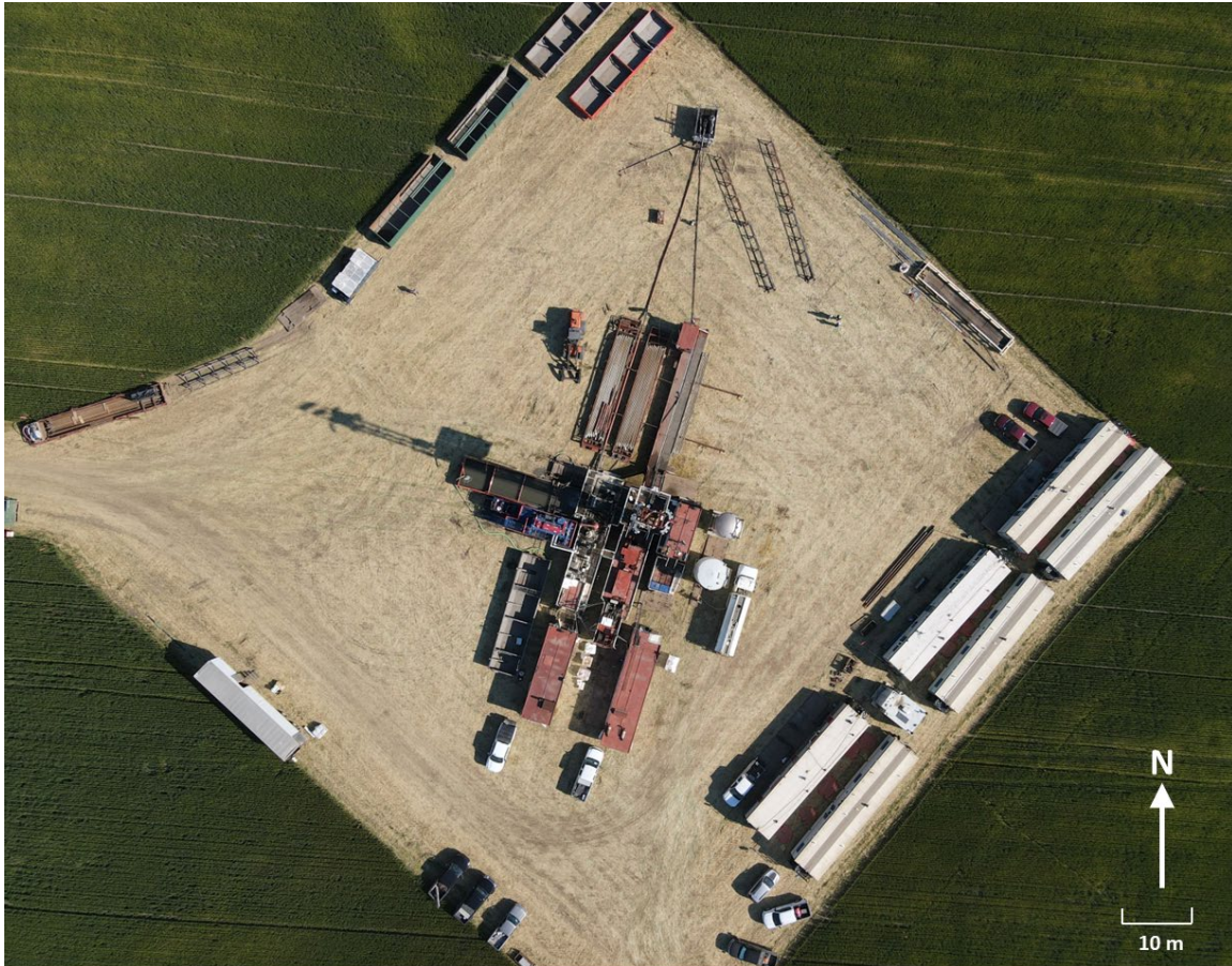
Figure 18-2: Constructed Surface Lease – Drilling Operation (GLC 102/04-15-032-23W3/00)
